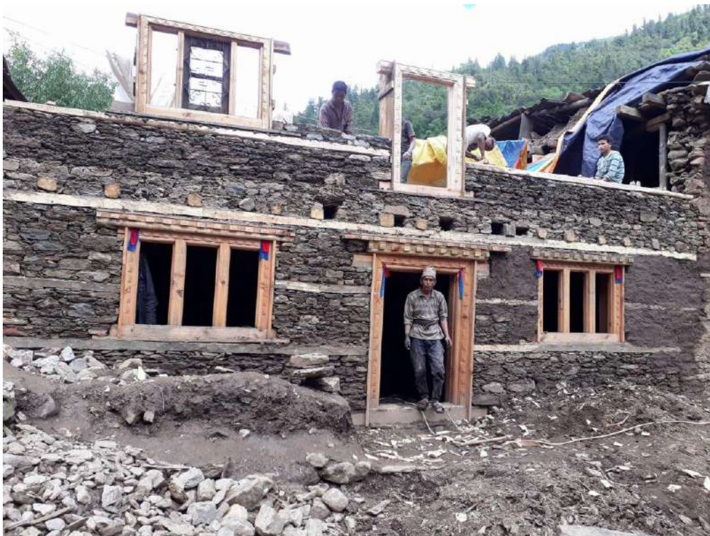
Figure 4 almost 50 percent monastery reconstruction work completed
