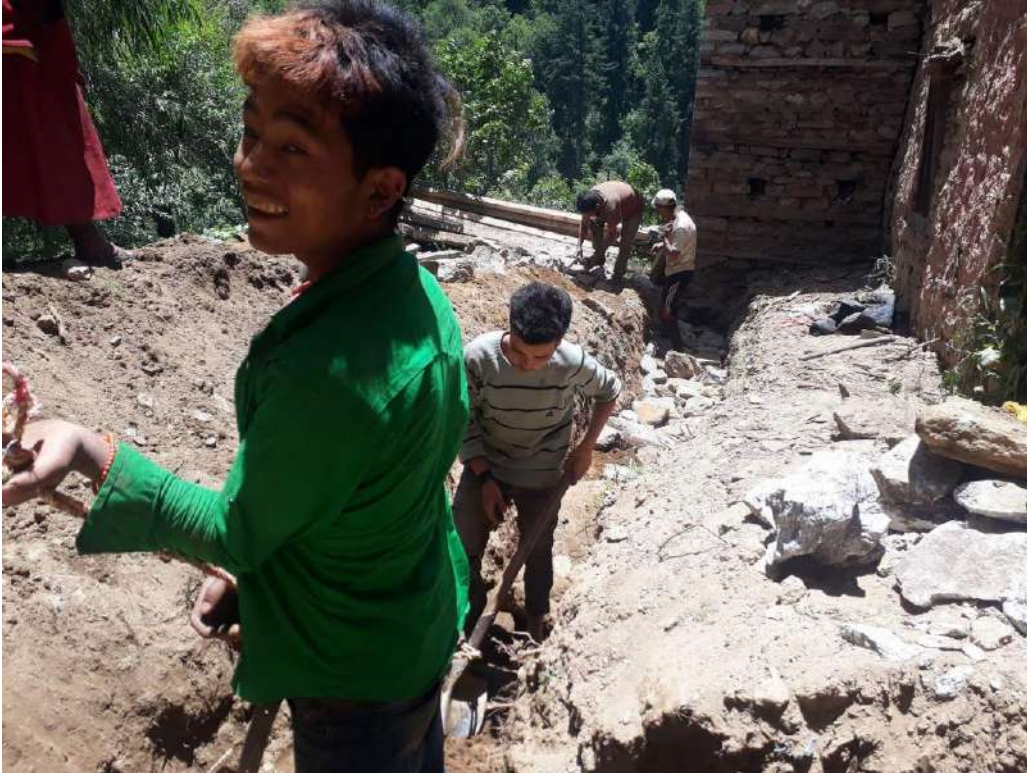
Figure 1 starting the monastery building foundation work
