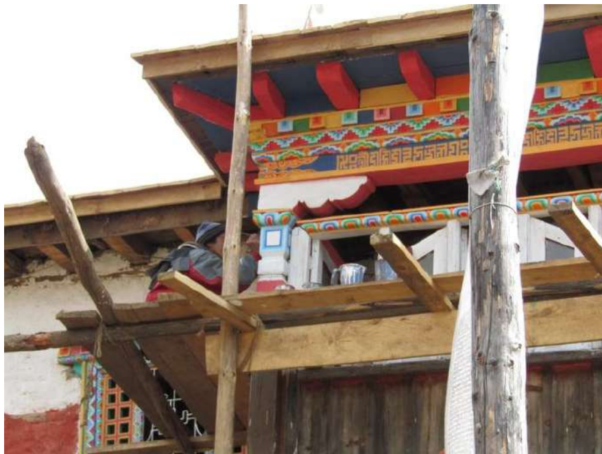
Figure 14 Painting work is under going
