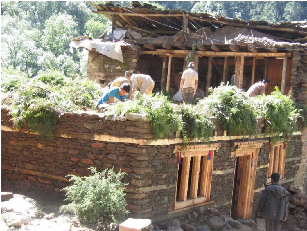
Figure 6 first floor completed
