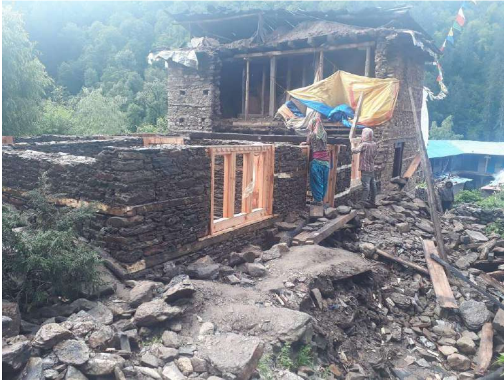
Figure 3 monastery building reconstruction is under construction
