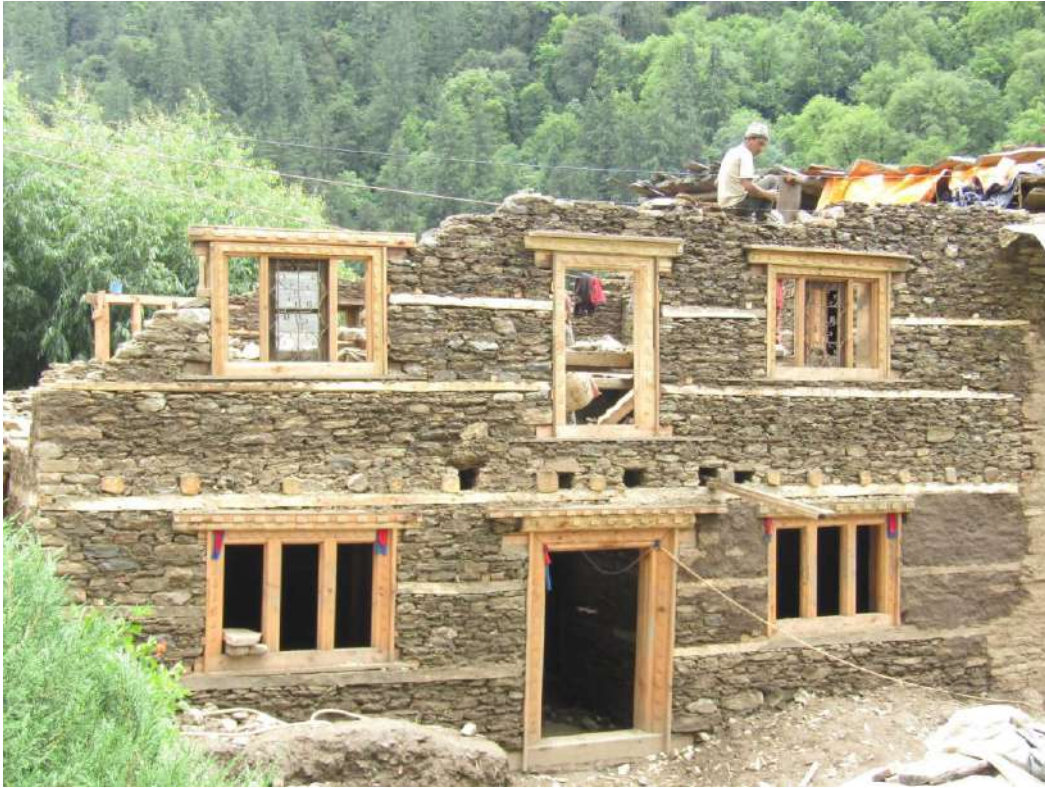
Figure 7 monastery building 75 percent completed
