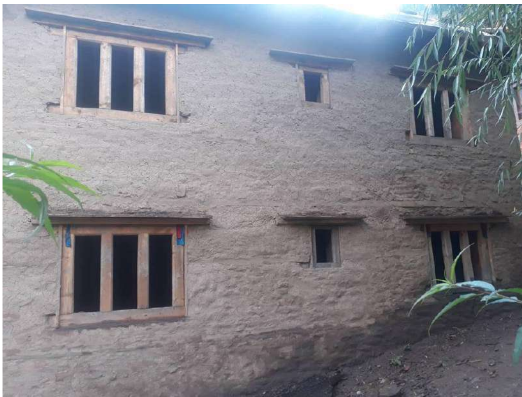
Figure 9 backside of the monastery building
