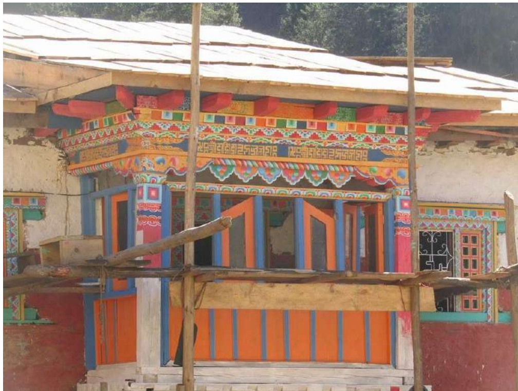
Figure 16 Wooden plank roofing
