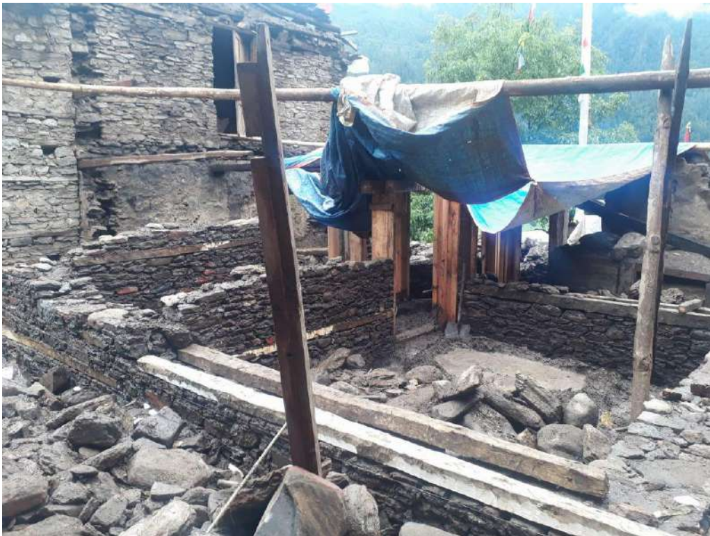
Figure 2 starting the building reconstruction project
