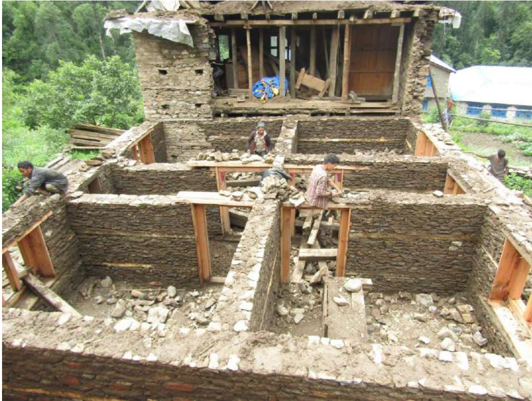
Figure 5 building is under construction
