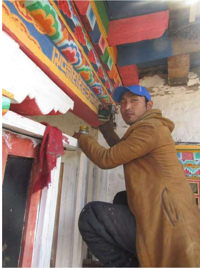
Figure 13 Painting work is under going
