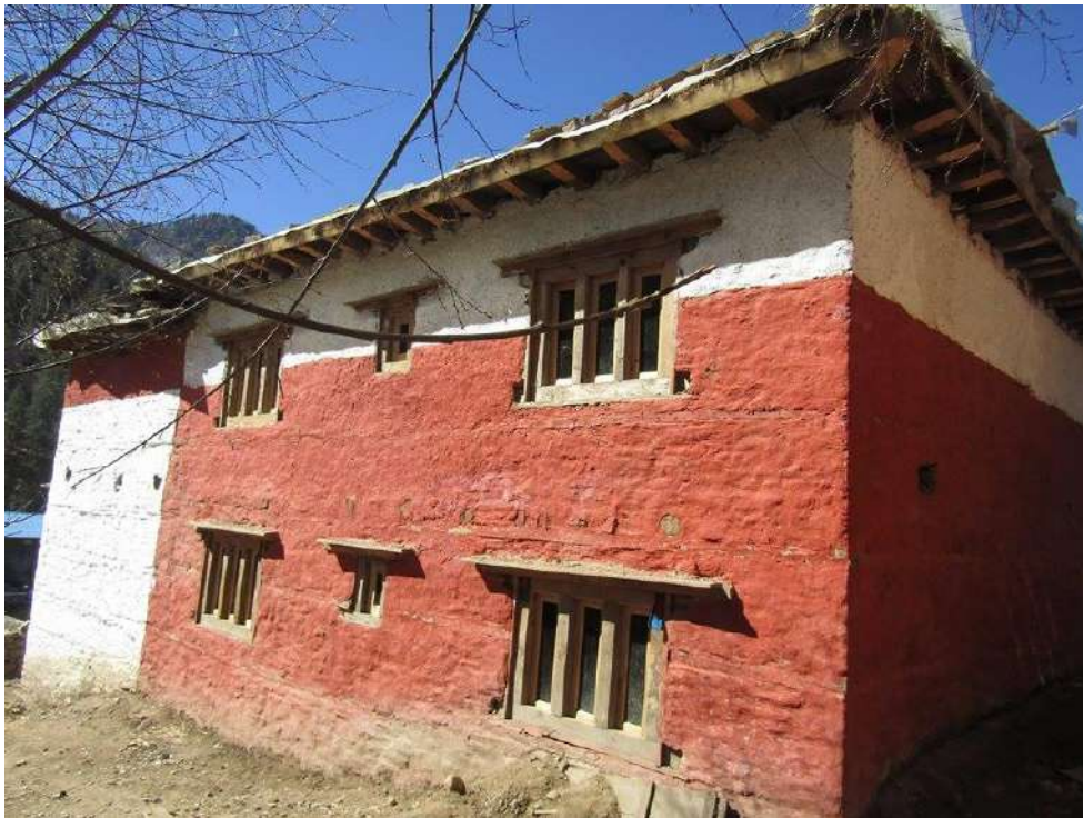
Figure 18 Final looks from back side of the monastery building
